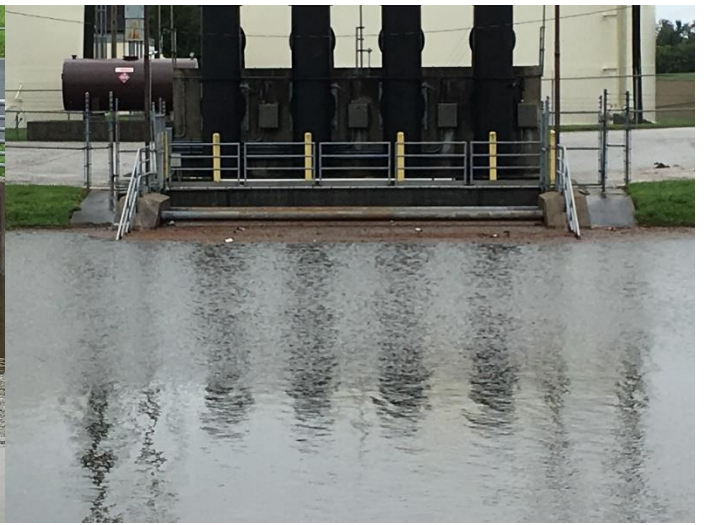
Approx. 5 ft freeboard within concrete pump box 4 x 22,000 GPM pumps
