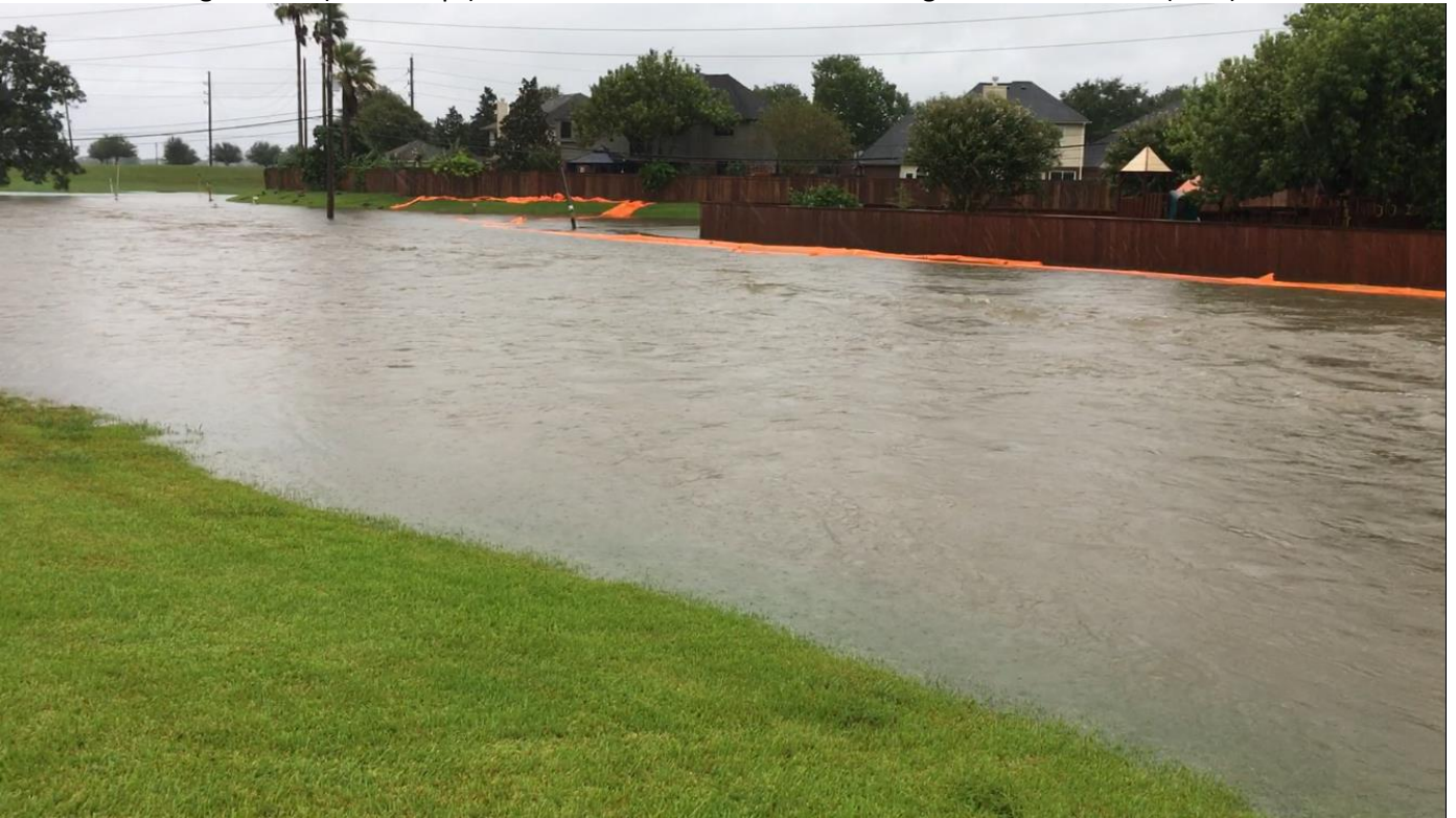
Commercial tract tiger dams at rain sourced high water – (Tue AM 8-29)
