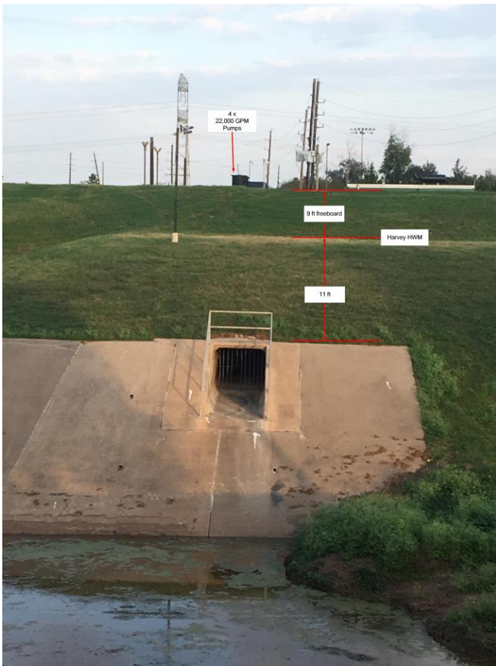
Pump outflow culvert was approximately 11 ft under water at the Harvey HWM.
