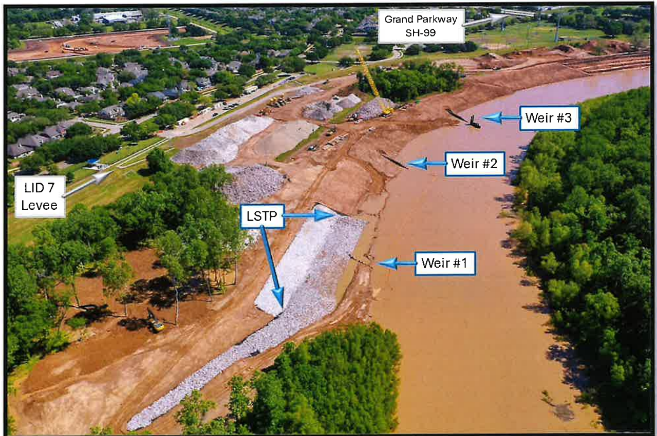
April 11 Construction Progress (prior to flooding)
